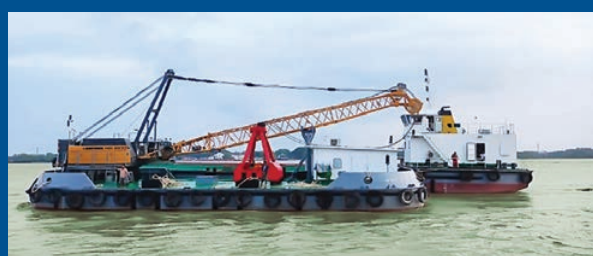
GDB-2 (26M Grab Dredger)
